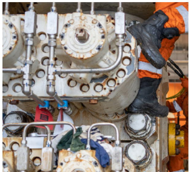
Deep-Water Bop Stack Services
